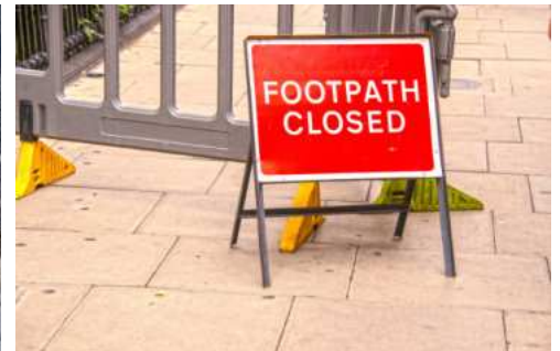
Roadworks blocking access
